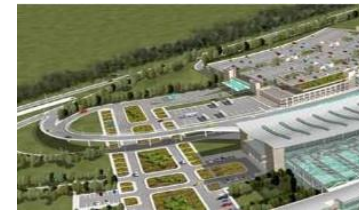
TAV, Esenboga Domestic-International Terminal and Car Park
