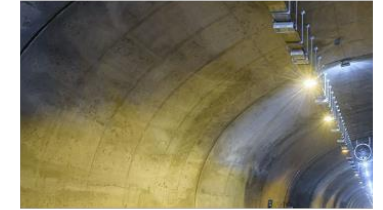
The Northern Marmara Motorway Project
