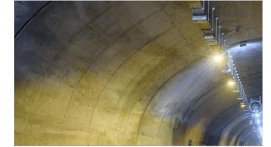
The Northern Marmara Motorway Project
