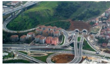
Seven Hills Seven Tunnels Project
