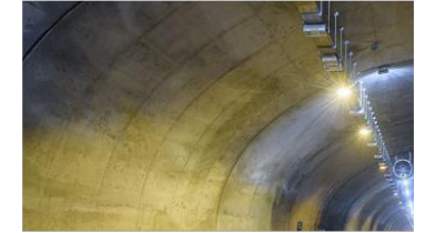
The Northern Marmara Motorway Project
