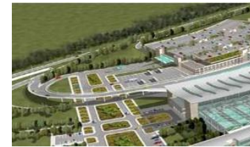
TAV, Esenboga Domestic-International Terminal and Car Park
