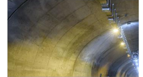
The Northern Marmara Motorway Project
