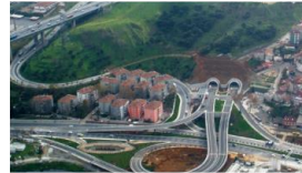
Seven Hills Seven Tunnels Project
