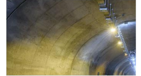
The Northern Marmara Motorway Project
