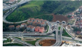
Seven Hills Seven Tunnels Project
