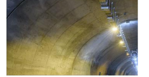
The Northern Marmara Motorway Project
