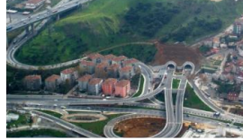
Seven Hills Seven Tunnels Project
