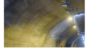
The Northern Marmara Motorway Project
